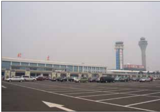
Das Project Beijing Airport Terminal 1 in China, Fertigstellung im Jahr 2004 The Project Beijing Airport Terminal 1, China, Completion Date in 2004
