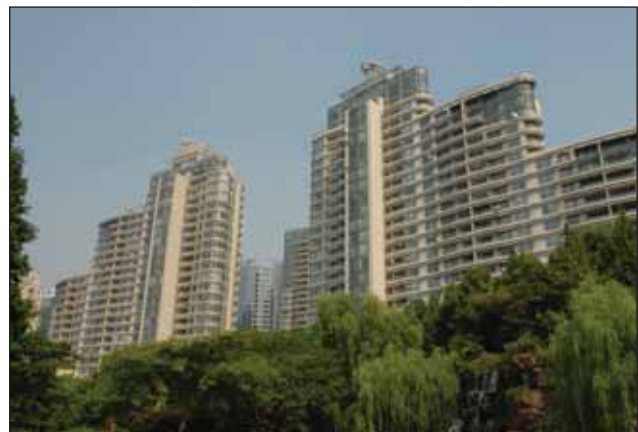
Project Top of City, ShangHai, P.R. of China, Project Apartments auf 245 m 2 Project Top of City, ShangHai, P.R. of China, Project Apartments at 245 sqm
